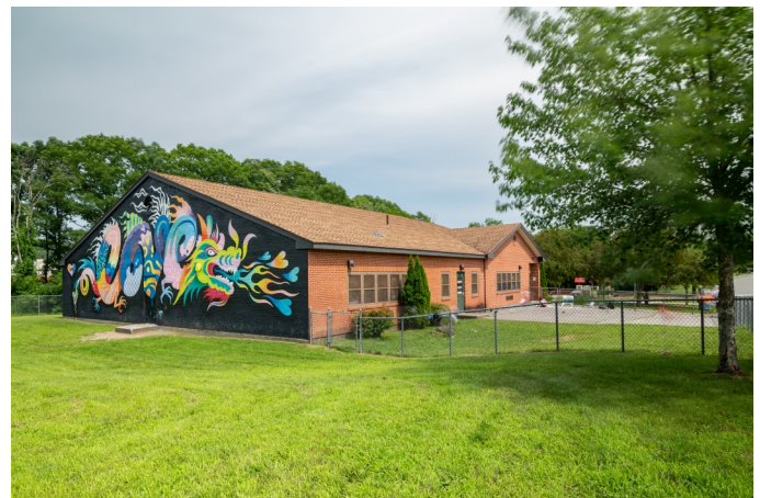
Current Club site located at 180 Constitution Ave.
